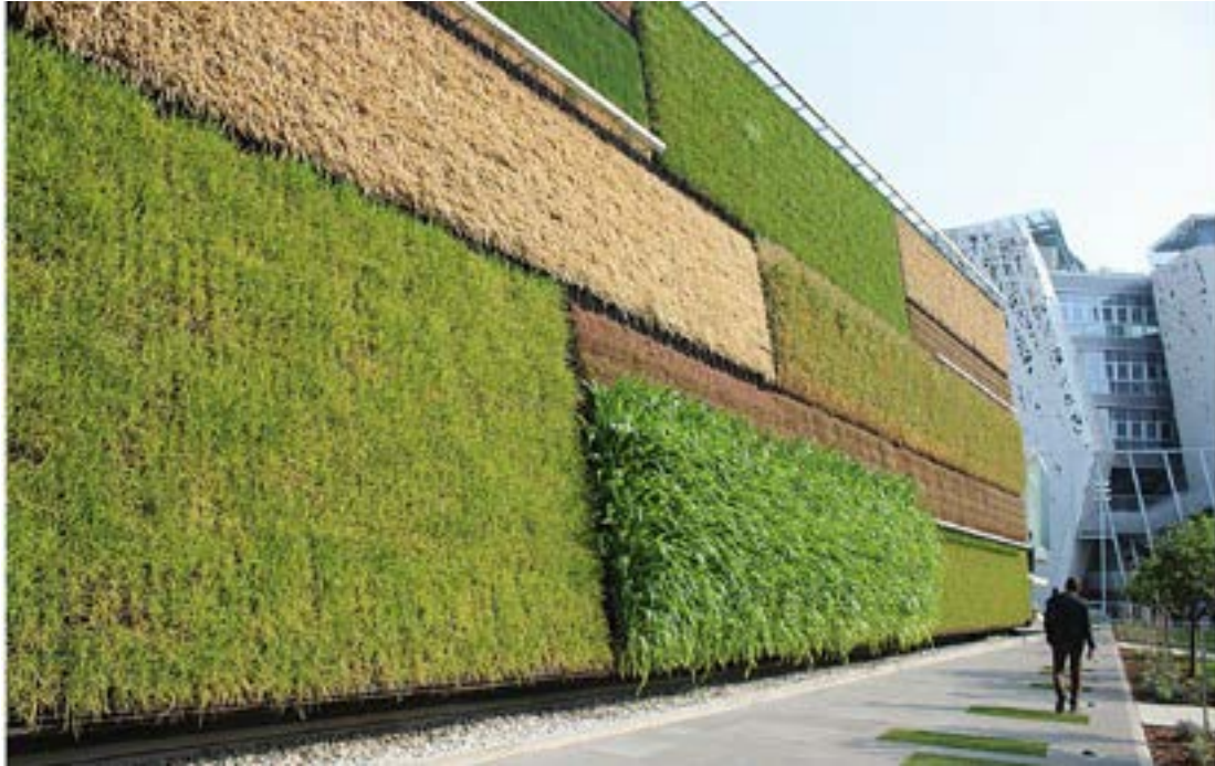
Figure 4: The Israel Pavilion's Vertical Field was built of Modular tiles set into a massive steel frame elevated above the ground, photo @ Claire Diebel
