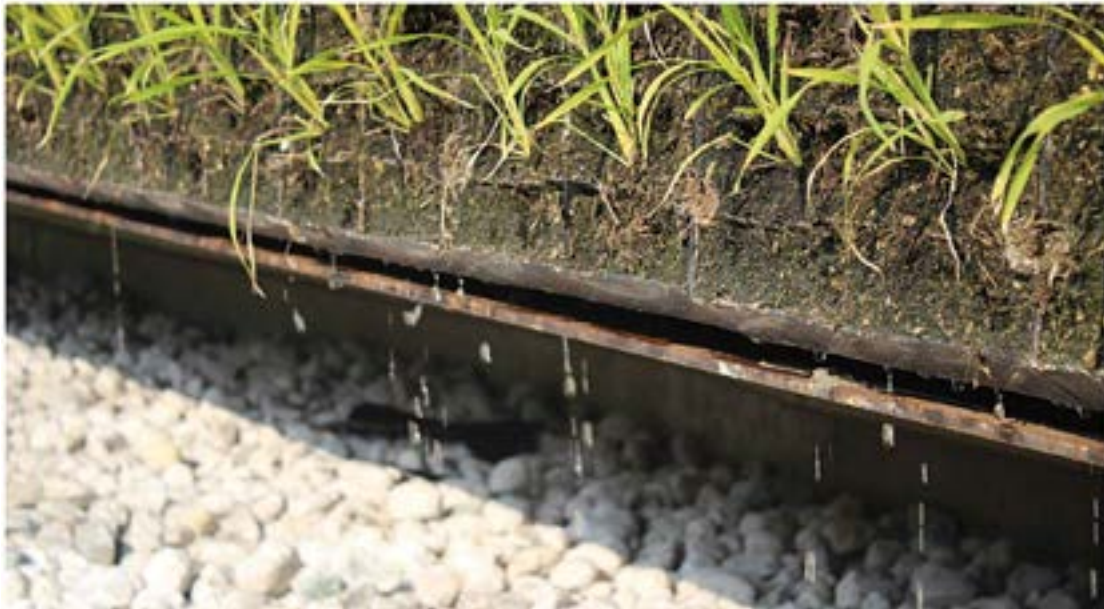
Figure 5: The drip irrigation was designed for excess water to exit the growing media, photo @ Claire Diebel
